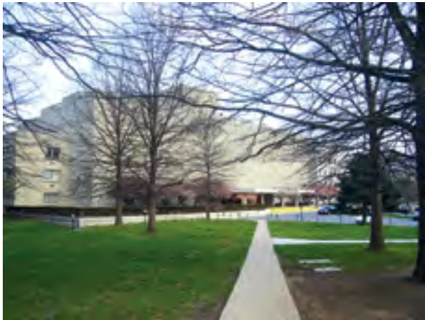
Fig. 8. The main building of AFIP
